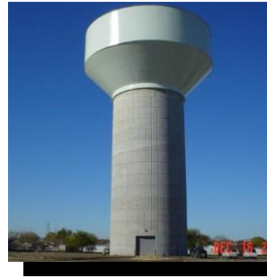
Water Delivery System Development
